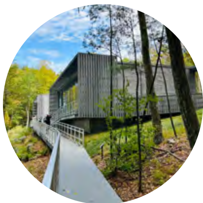
Alford Coastal Research Center, Newbury, US (Flansburgh Architects, 2022)
